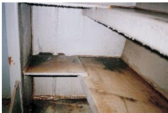
Figure 6.5 Viable microbial biofilms adhering to cargo tanks before biocide decontamination
