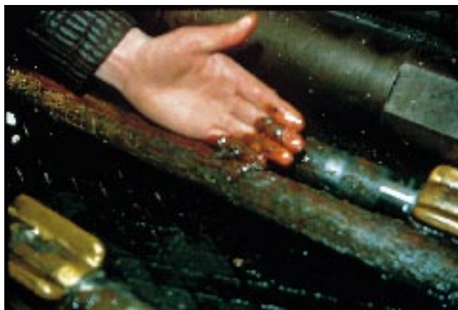
Figure 2.12 Microbial slime in hydraulic oil system
